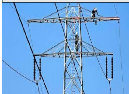
Extra belasten (40 MW)
